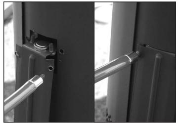
Figure 55: Spill switch installation.
