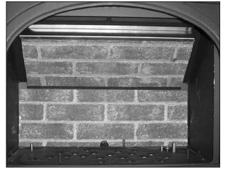
Figure 69: Back brick panel in place.
